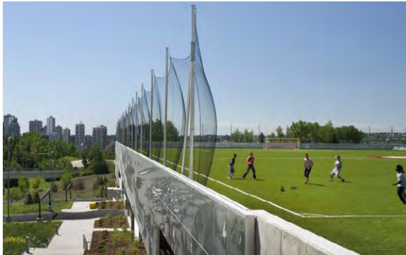
PARKADE UNDER COHOS COMMONS FIELD, SOUTHERN ALBERTA INSTITUTE OF TECHNOLOGY
