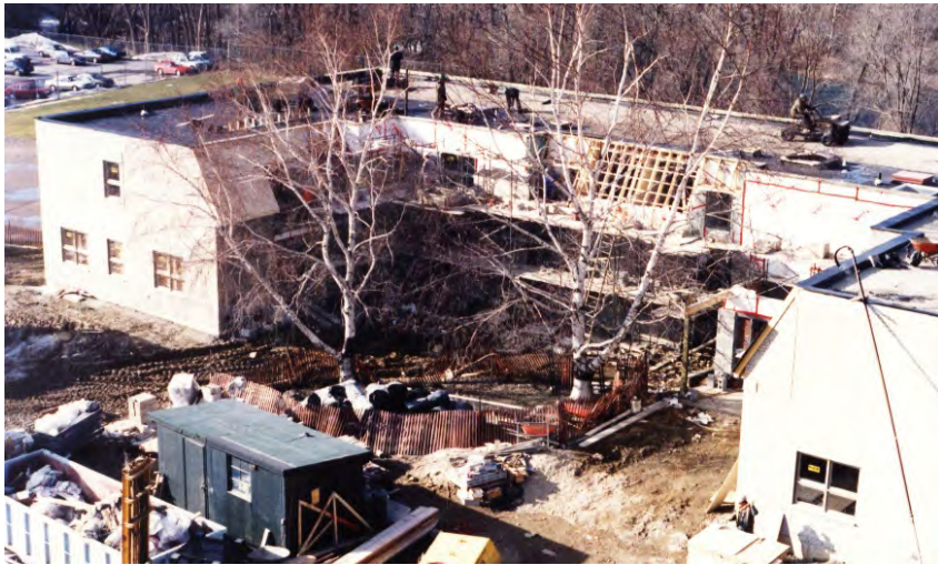
FIGURE 6. CONSTRUCTION OF ALUMNI COURT HOUSING / 1990
