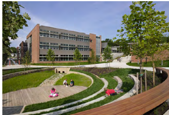
OURDOOR CLASSROOM, MANASSAS PARK ELEMENTARY SCHOOL, VIRGINIA
